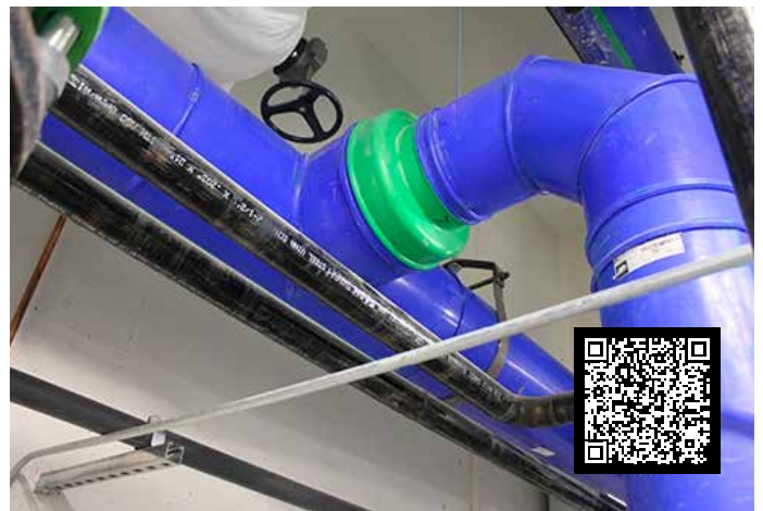
PROJECT Bozeman Health Hospital
